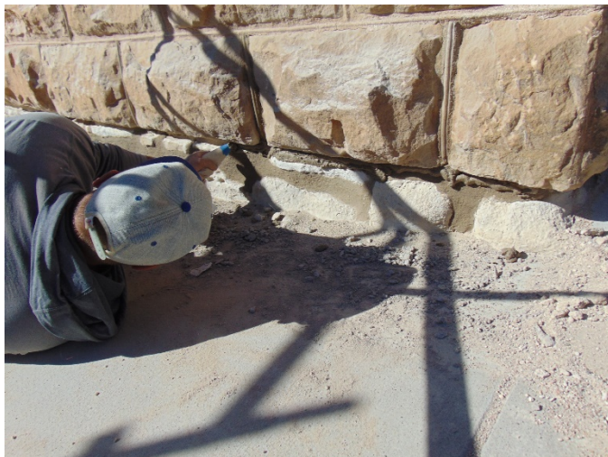
Mountain Masonry repairing the foundation
